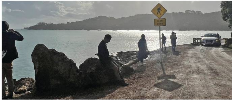
In 2010 the Esplanade was closed due to safety concerns and then reopened a year later. After a later review, Auckland Transport concluded that the road was too degraded to be safely driven on. Photo Sarah Gloyer
